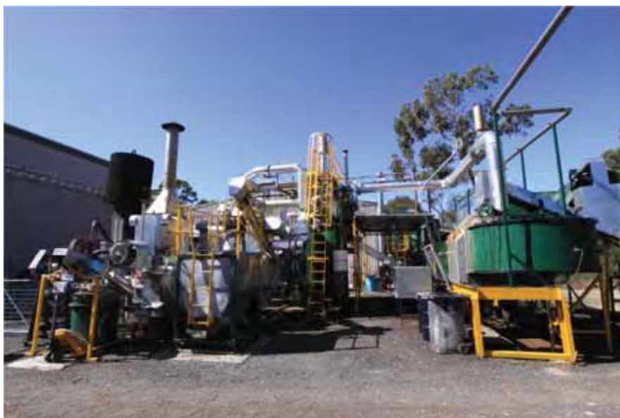
Figure 3: Pacific Pyrolysis Pty Ltd's slow-pyrolysis demonstration facility at Somersby, Australia. Production facility for Agrichar™ biochar and bio-electricity from syngas.
